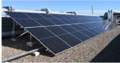
Photovoltaic generation (4x15kWp)
